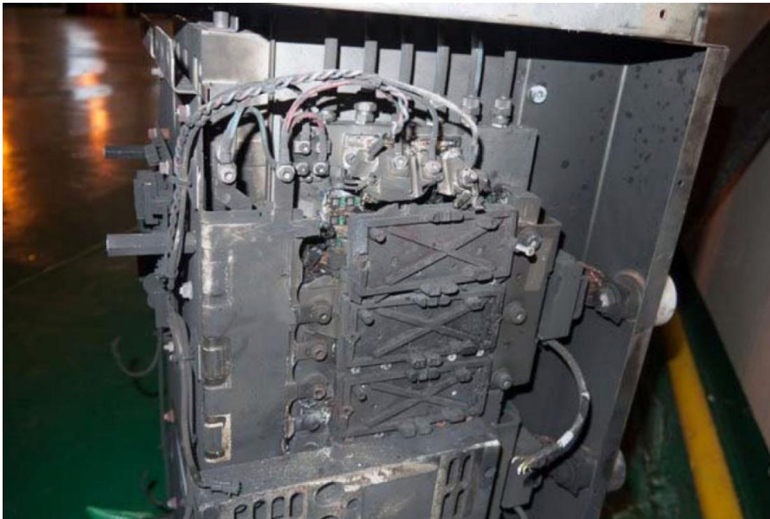
Fig 22 : Result of common mode voltage interference on 3MW PWM VFD
